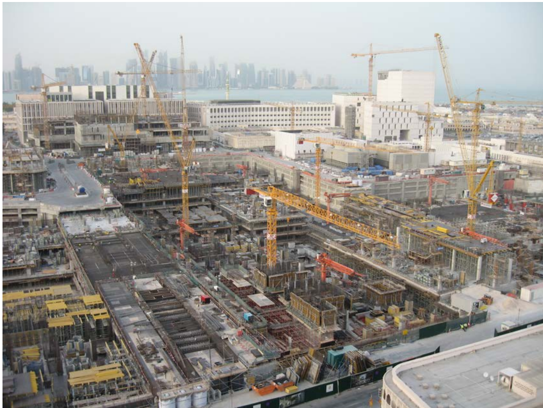
Figure 3. Msheireb downtown redevelopment construction site in December 2013. Source: Author.
