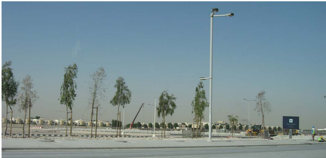
Figure 5. Trees at the Lusail construction site, December 2013. Source: Author.
